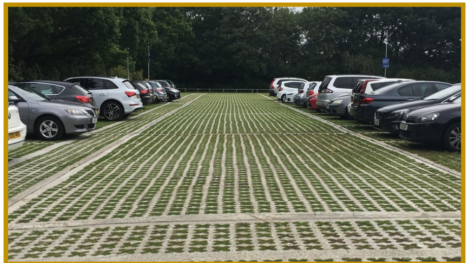
Figure 39: Grass Concrete Pavers
