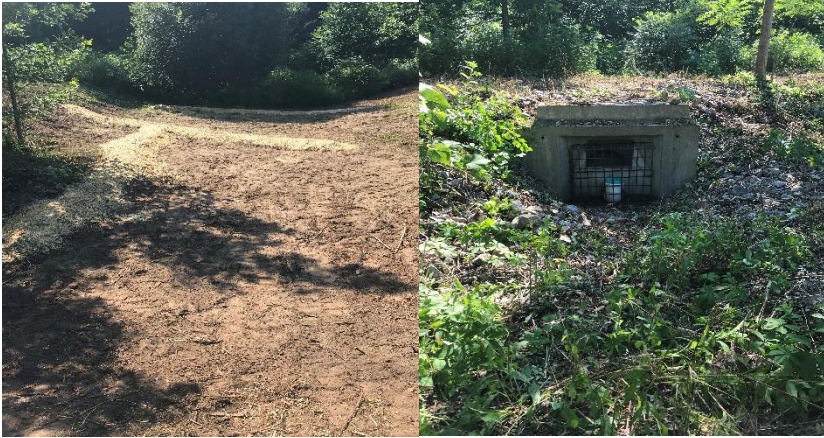
- Hawthorne Road Lat 41.5946 Long -72.4935
