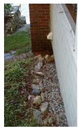
**Installation**: Dig a trench that is 18" wide and at least 8" deep along the drip line. Slope the bottom away from the house so that water will drain away from the foundation. Make sure to dispose of the soil in a flat area where it cannot be washed into the lake. Fill the trench with  $\frac{1}{2}$ " -1\frac{1}{2}" crushed stone. The front and sides of the trench may be edged with stone or with pressure-treated lumber to hold the stones in place.
