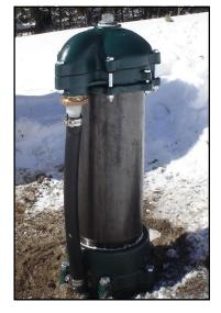
A typical water supply wellhead consists of a cap and seal, as well as an air vent. East Hampton relies primarily on private wells on individual properties.
