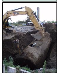
Removing Underground Storage Tanks is essential to protecting groundwater resources.
