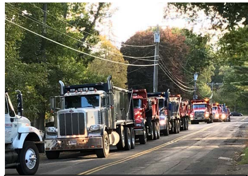
Contractor crews delivering asphalt to Sunset Drive today.
