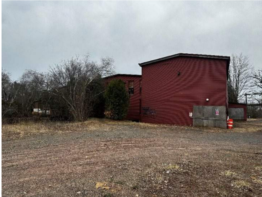
View of Northeast side of building, looking southwest
