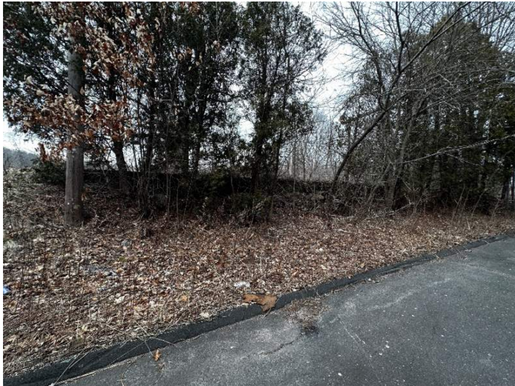
View to the north from westernmost side of building, former building foundation. Transformer pad to the right in the photograph.
