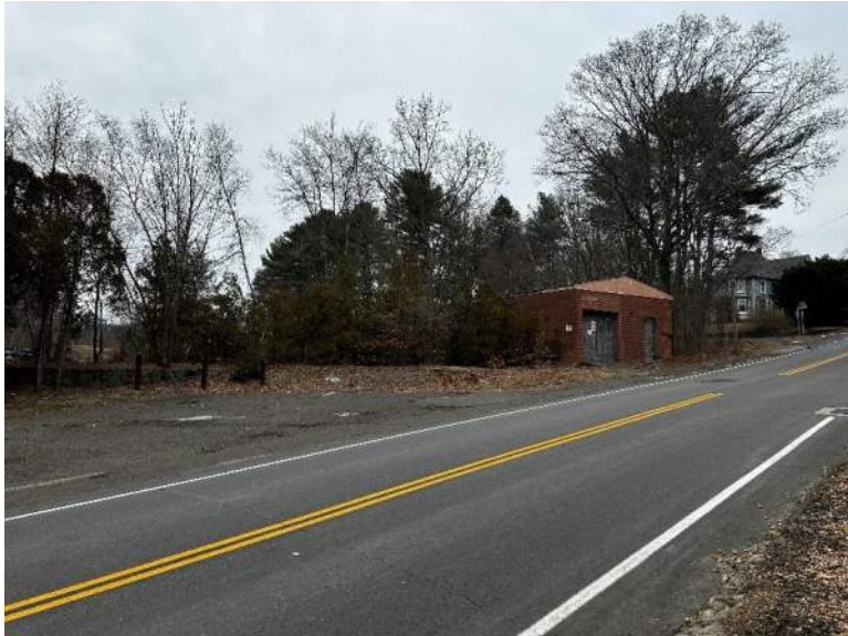
View of gate house looking northeast from Summit Street.
