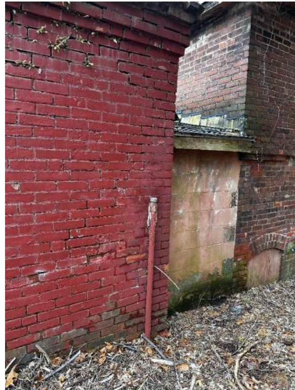
UST fill pipe east of former fire pump house
