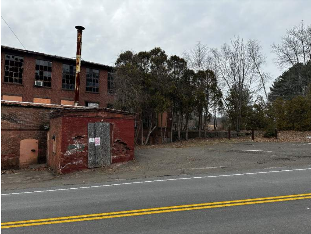
Views of southern side of building along Summit Street. Fire pump building in forefront. Second Pond to the right. Fill pipe and potential 3,000-gallon heating oil UST to the right of the pump building.
