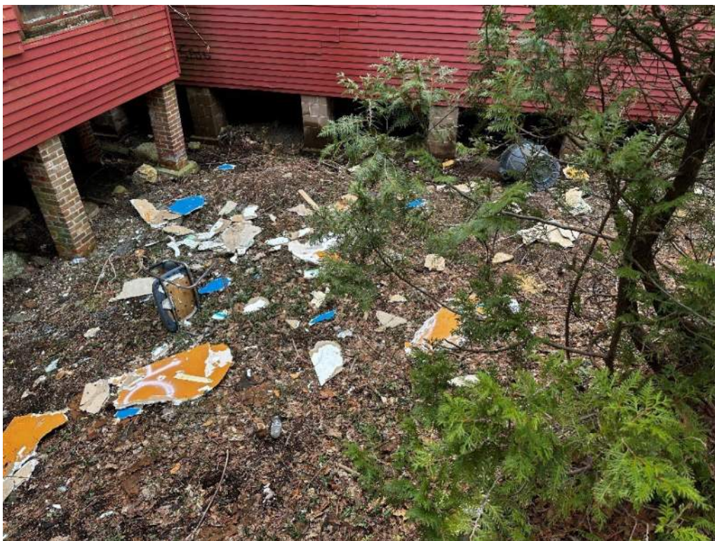
Northern side of building.
