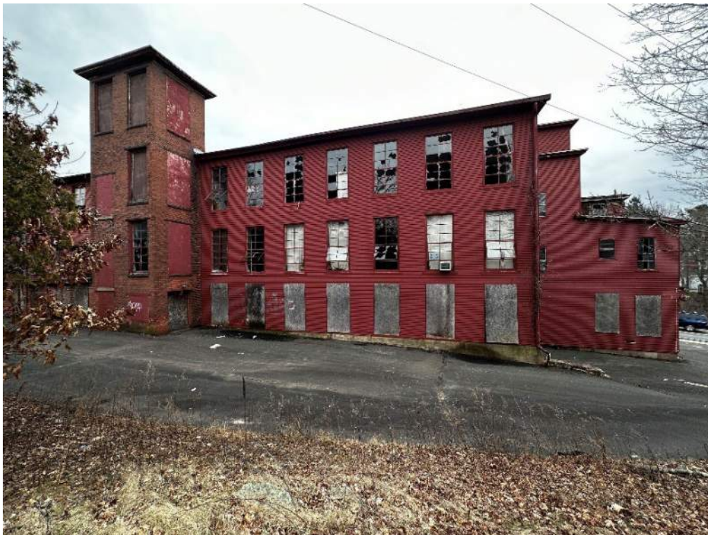
View of westernmost portion of building, looking south. Multi-level elevator shaft.
