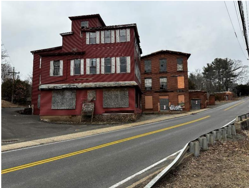
View of southwest corner of building. Portion of building contained office, elevator, heating oil AST, water wheel, tail race for the Pond runs beneath the building, under Summit Street to Pocotopaug Creek on the right side of photograph.
