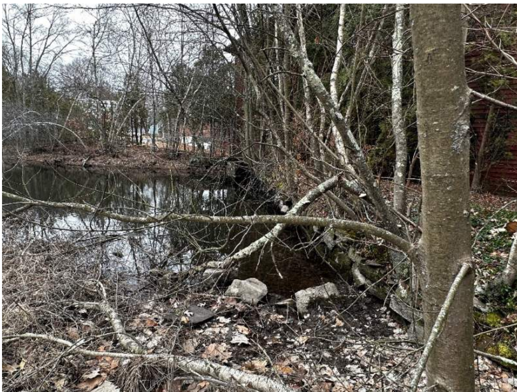
Western side of Second Pond as it enters beneath the building.
