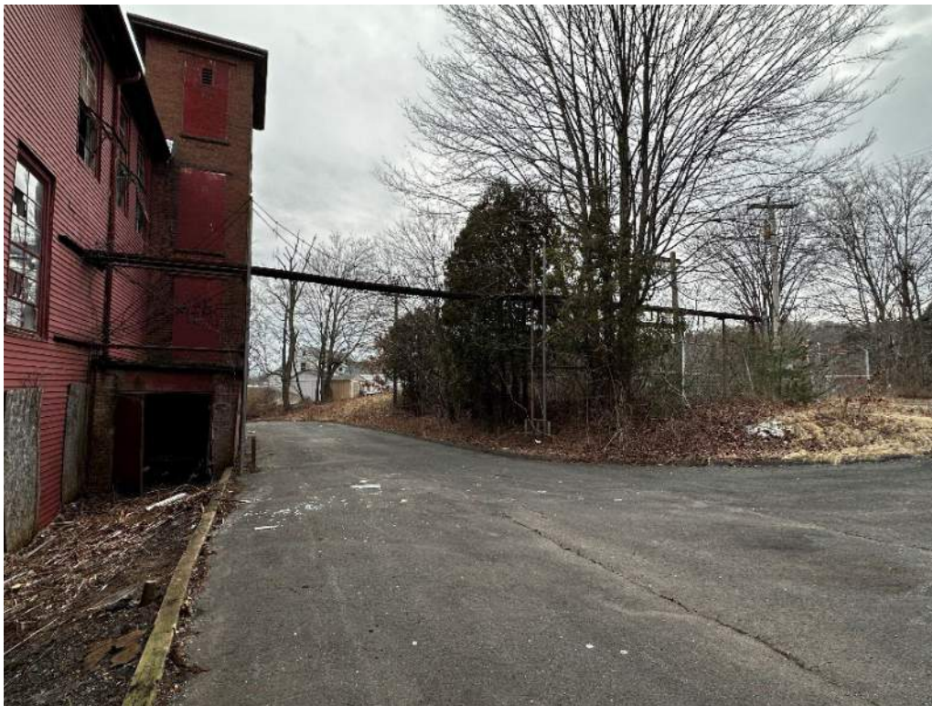
Overhead powerline trestle from building to transformer pad, located on north side of building. Multi-story elevator shaft in the rear.
