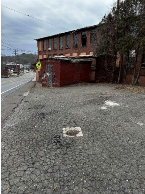
Monitoring well northeast of former fire pump house
