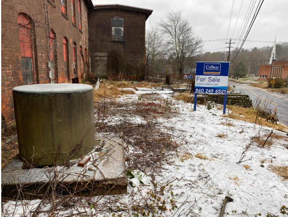
7: View of north side of building along Summit Street. Concrete pad behind "For Sale" sign was the location of the former Water Tower. Concrete structure in foreground in unknown and may have been access to a subsurface water tank.
