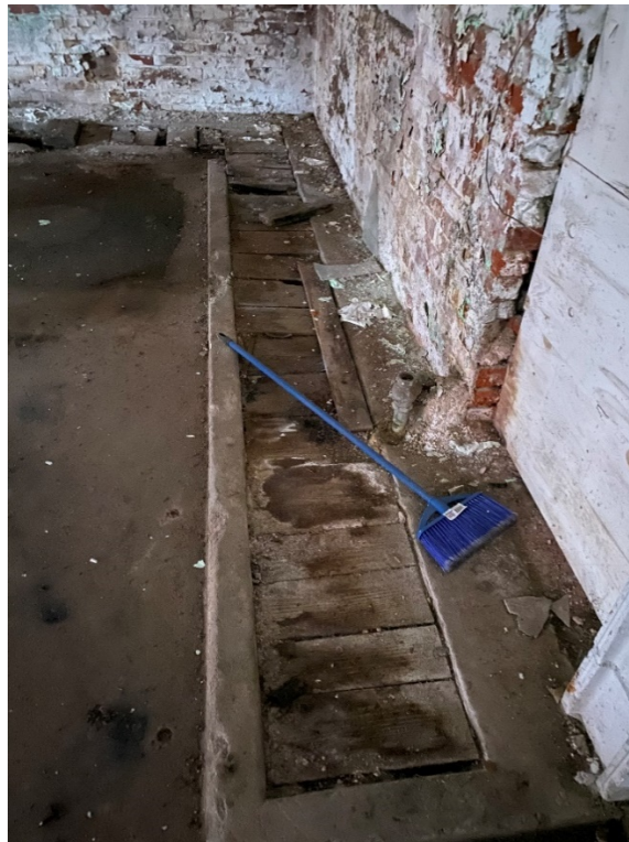
44: View of 1 st -story floor with manhole and floor drains.
