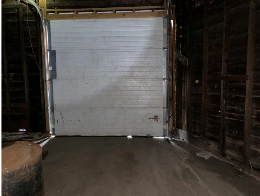
33: View of 1 st -story loading dock at southern portion of building.
