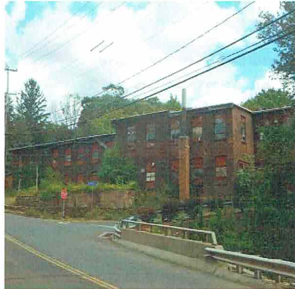
Site Photograph (September 2015)
