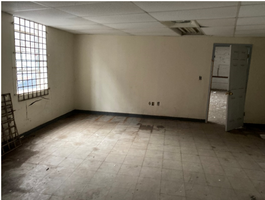
40: View of 1 st -story office with tile floor.
