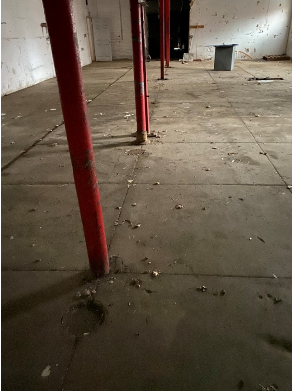
37: View of 1 st -story floor with manhole and floor drains.
