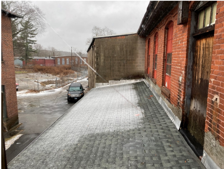
11: View of eastern side of building (roof of 1-story loading dock)
