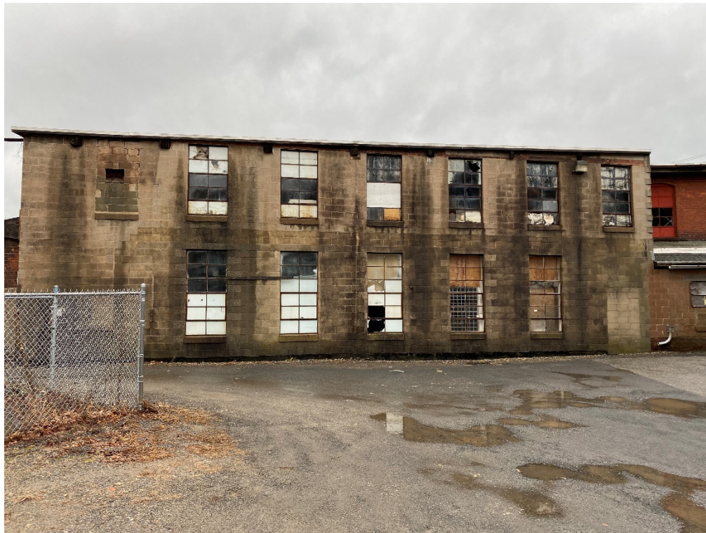
14: View of eastern side of building
