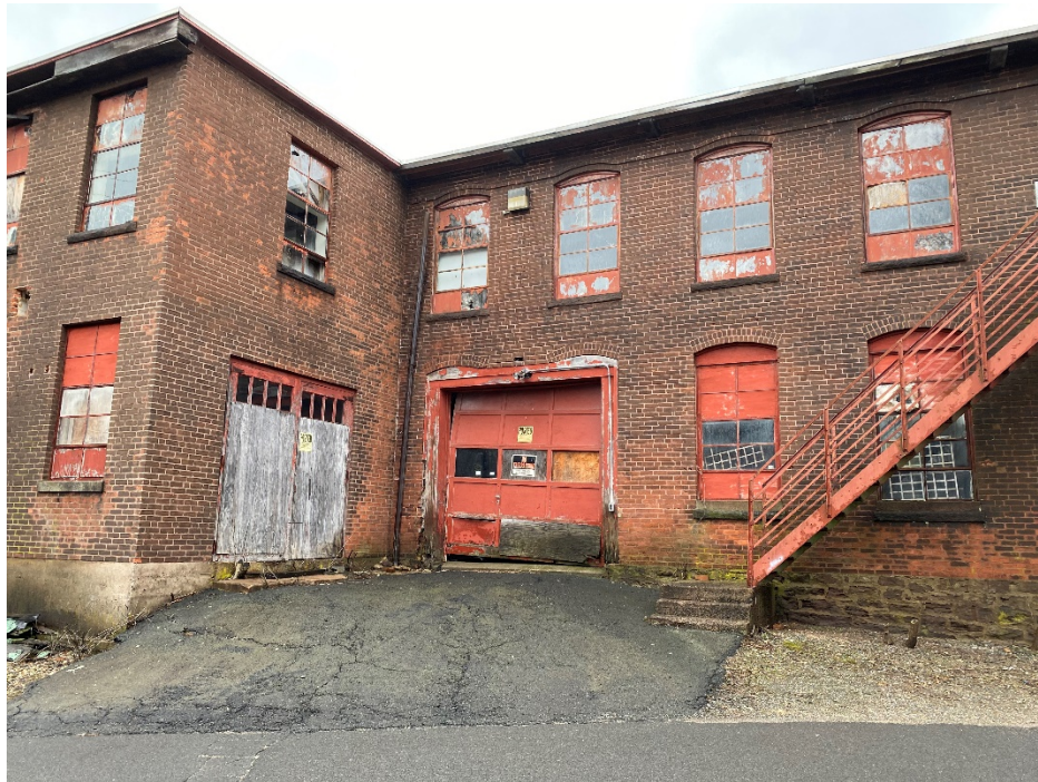
20: View of southwestern side of building, along Watrous Street
