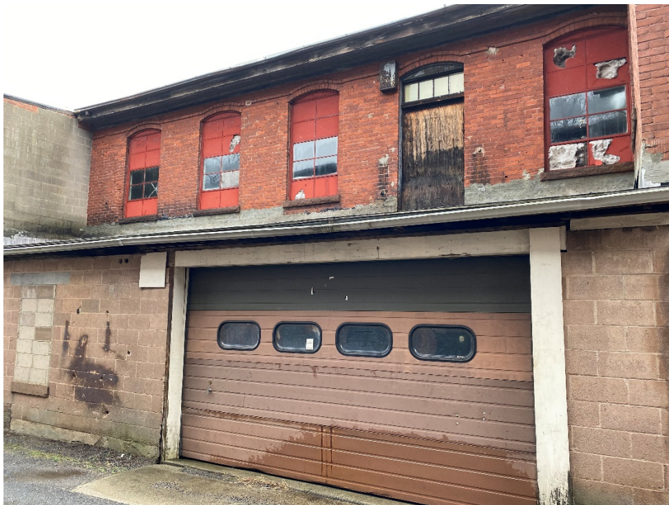
12: View of 1-story loading dock, eastern side of building
