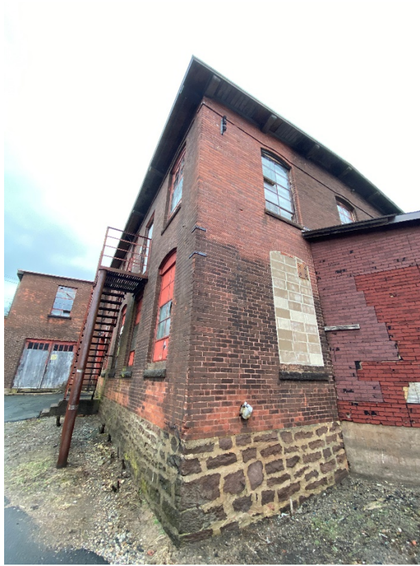
19: View of southwest corner of building
