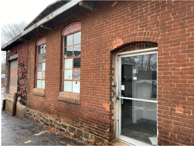
17: View of southern side of building
