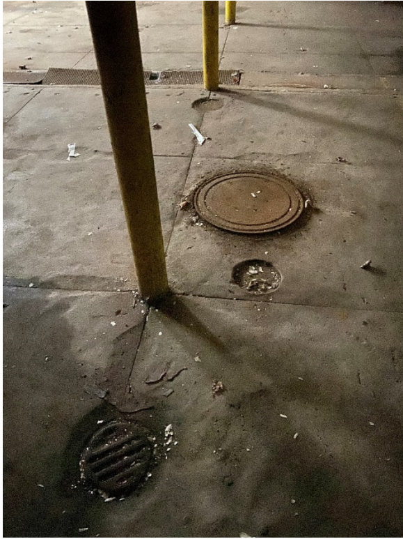
39: View of 1 st -story floor with manhole and floor drains.
