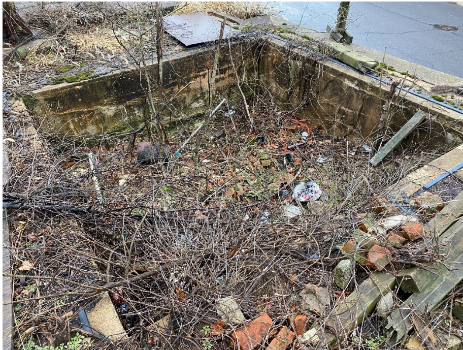
9: View of location of former Water Tower on north side of building.
