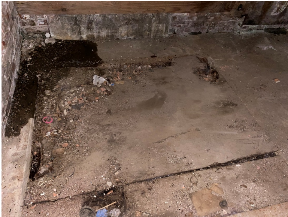
42: View of 1 st -story metal covered floor, northeastern portion of building.
