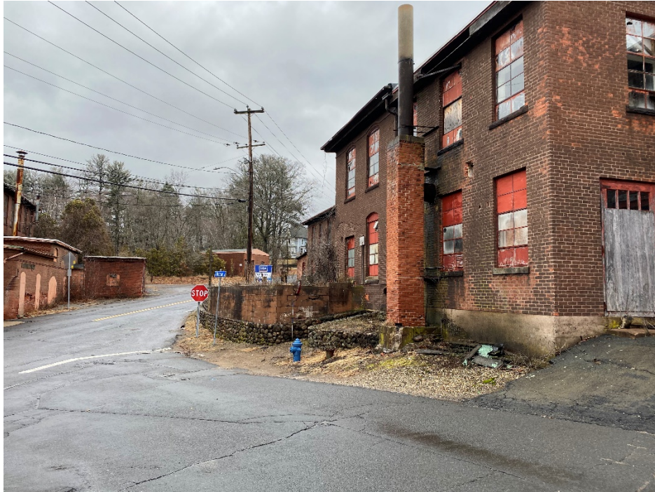
21: View of southwestern side of building, along Watrous Street
