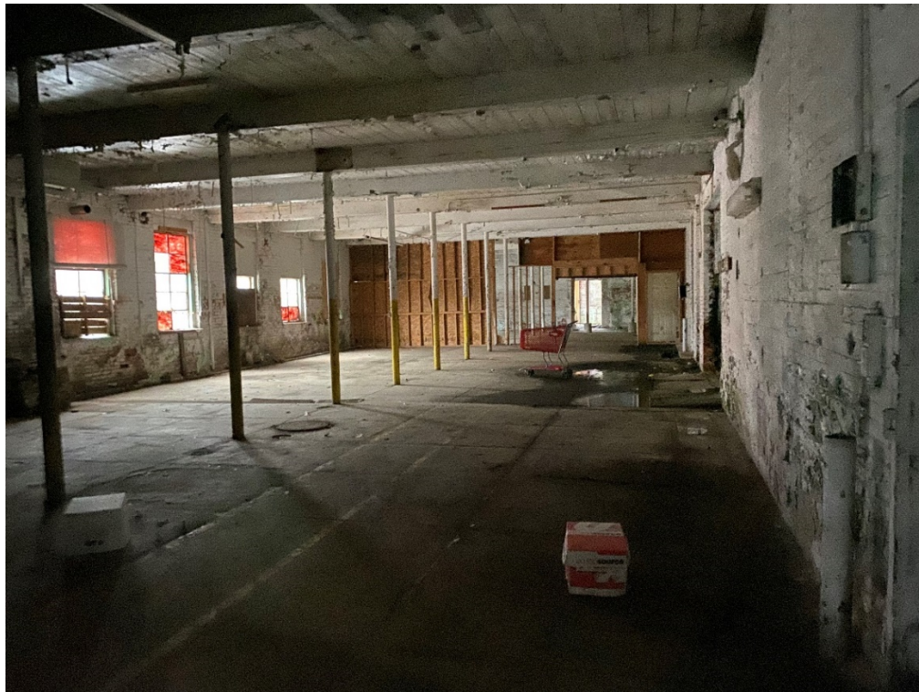
38: View of 1 st -story room, northern portion of building.
