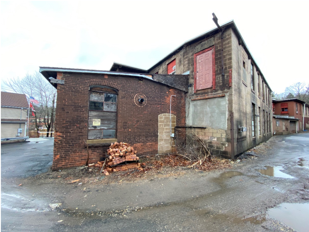
18: View of southeastern corner of building
