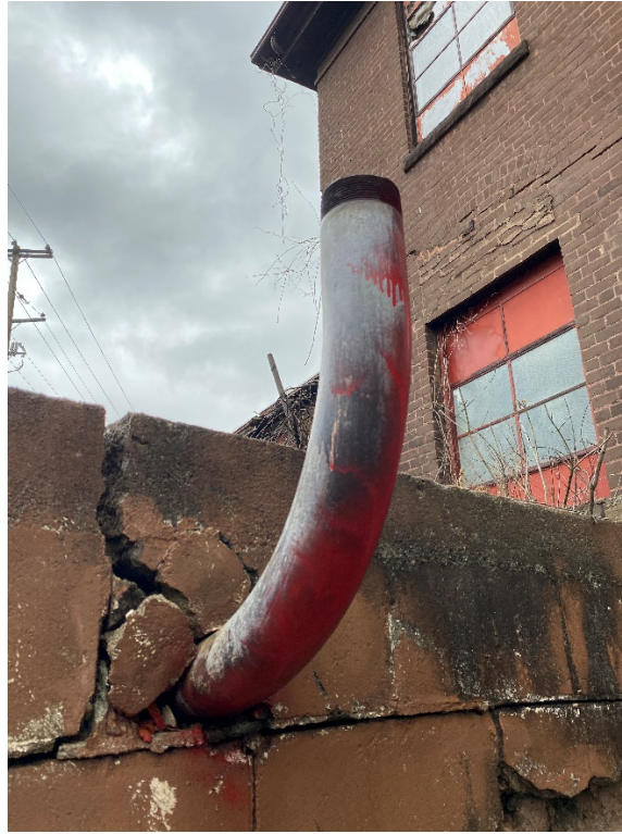
5: Fill or vent of apparent underground storage tank, corner of Watrous and Summit Streets.
