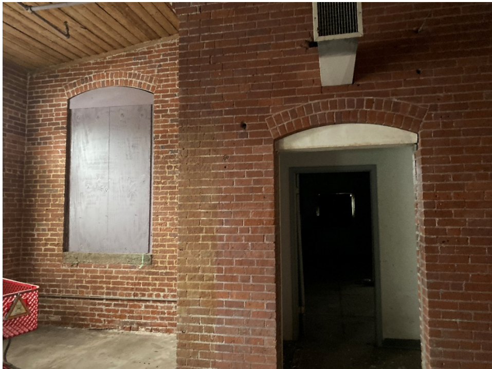
28: View of room at entryway on the southernmost portion of building.
