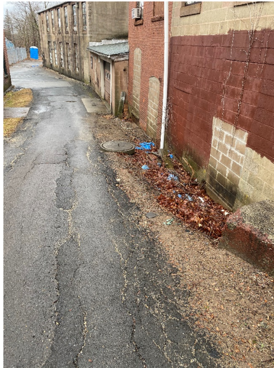
13: View of eastern side of building
