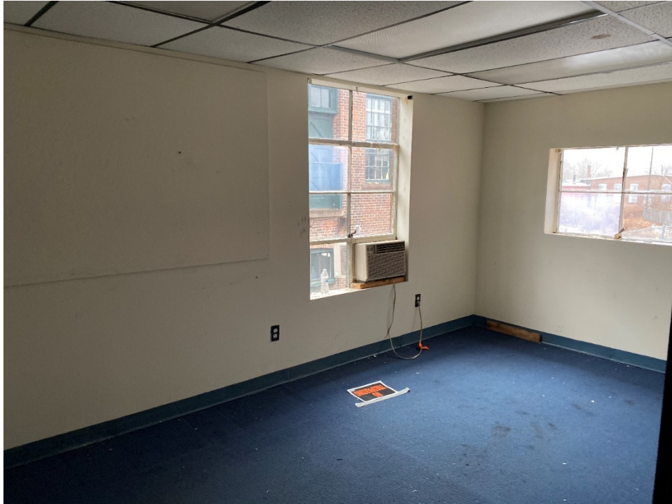
53: View of 2 nd floor office.
