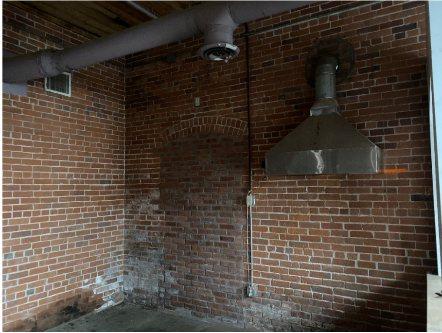
27: View of room at entryway on the southernmost portion of building.
