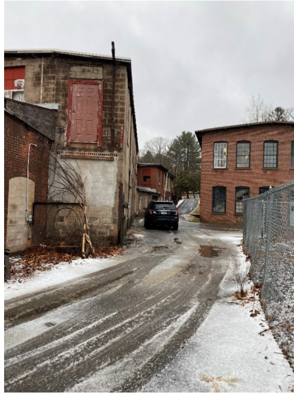
15: View of southeastern side of building
