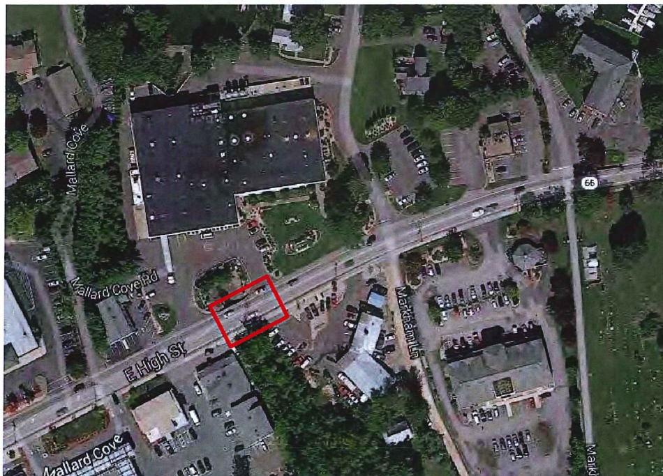
Aerial photo of Bridge No. 02018 and surrounding area (Google)
