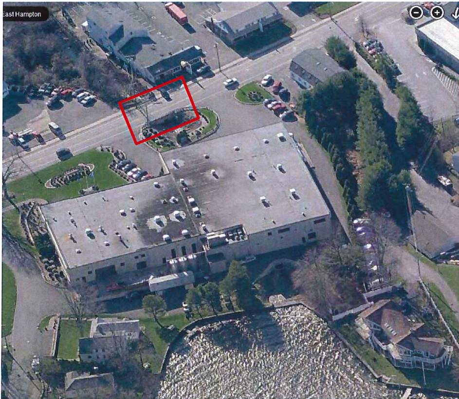
Birdseye aerial of Bridge No. 02018 Route 66 (East High Street) over Pocotopaug Creek looking southward. Pocotopaug Lake is visible at the bottom of the photo (Bing).
