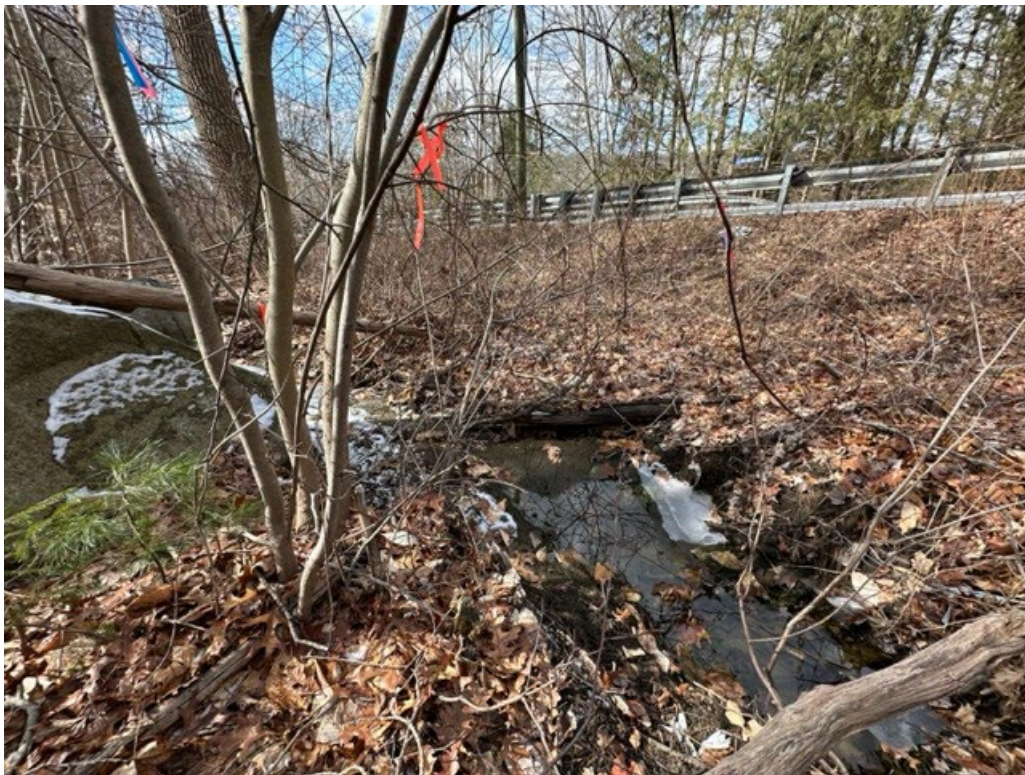
Photo 2: Example of the watercourse channel conditions along the road
