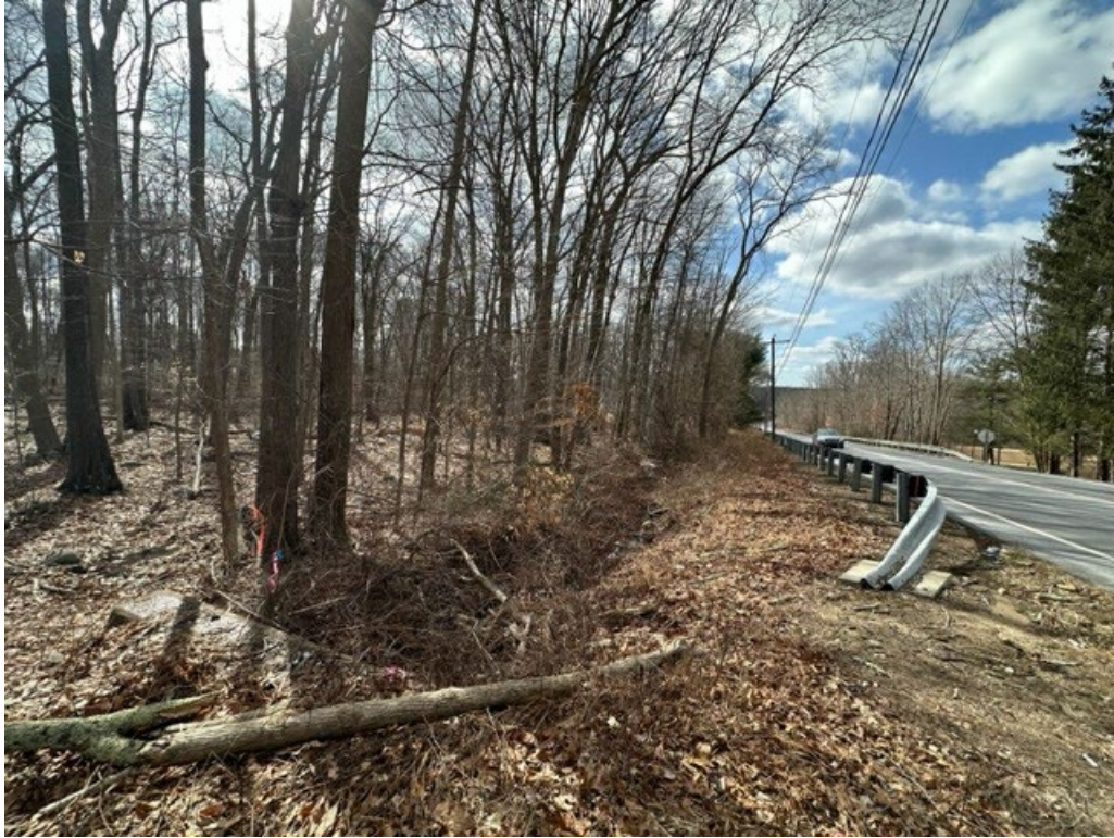
Photo 1: Drainage that runs along the road frontage.
