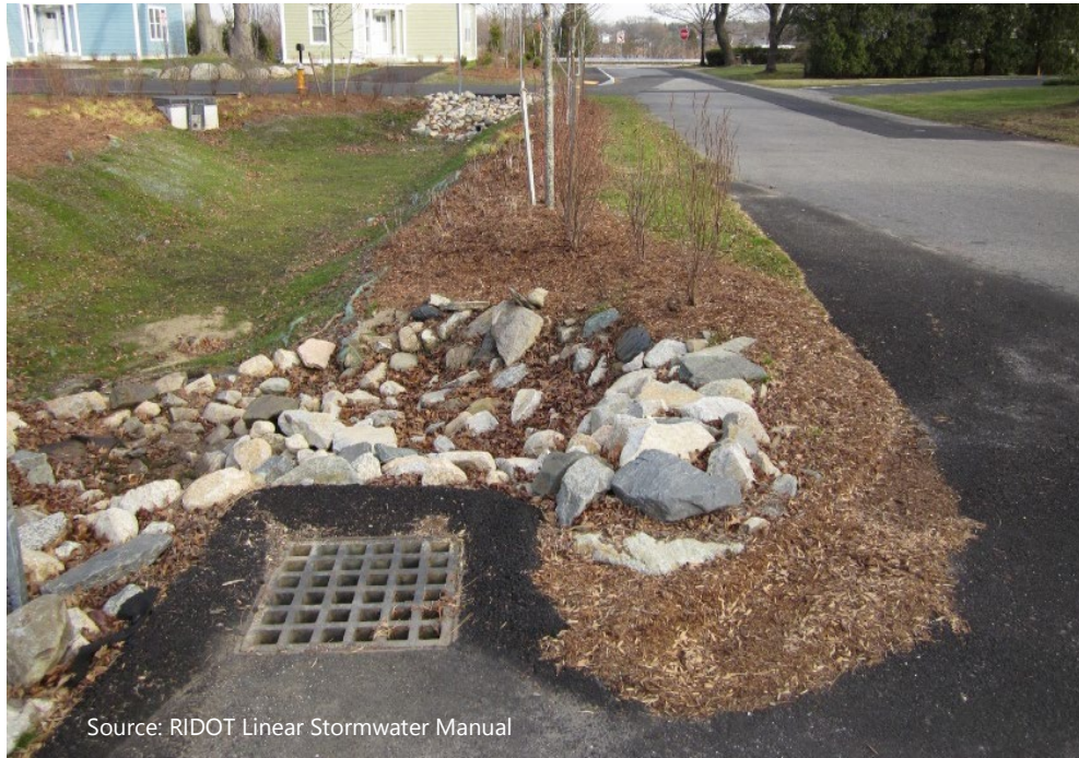
Figure 13-40. Deep Sump Catch Basin Inlet Structure
