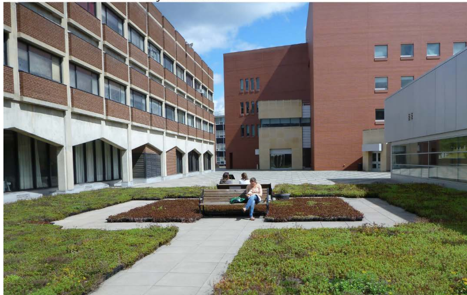
Full Roof with Modular Tray Installation
