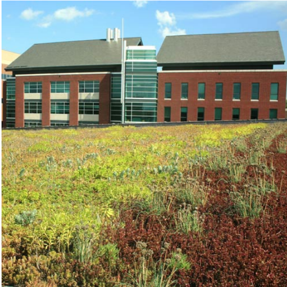
Extensive Green Roof, Laurel Hall, Storrs, CT
