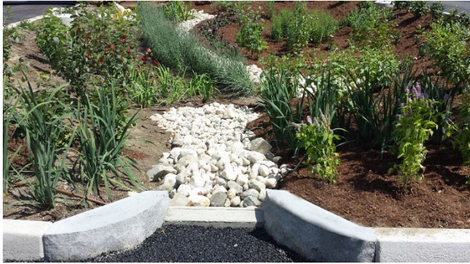
Curb cut openings at inlets to bioretention basins designed to capture runoff from adjacent parking areas.
