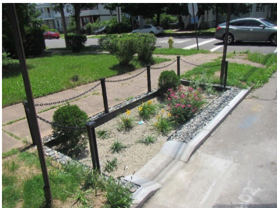
Roadside bioswale in urban residential setting.
