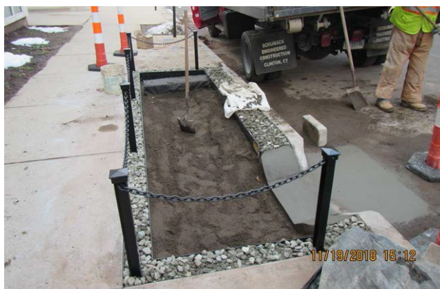
Installation of depressed concrete pad in front of inlet curb opening to create a low point that helps convey gutter flow into the bioswale (left photo). Curb cut opening to direct road runoff beneath the adjacent sidewalk into a stormwater BMP (right photo).
