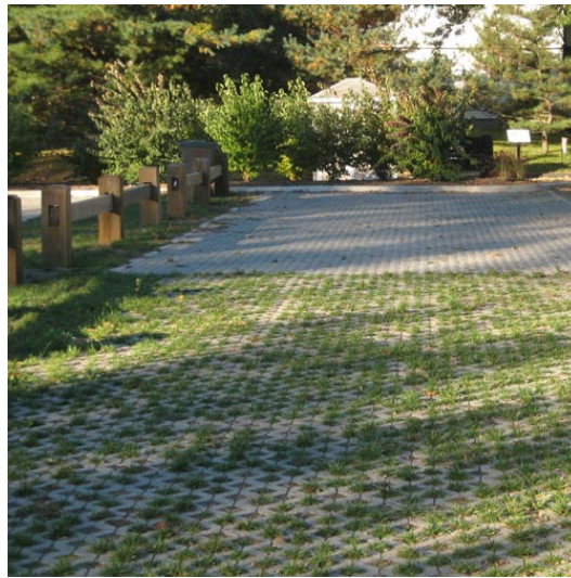
Grass and Grid Pavers (Hole in the Wall Parking Lot, East Lyme, CT)
