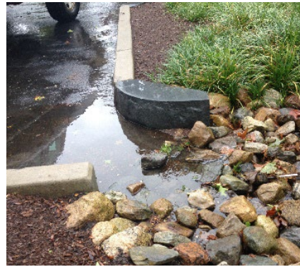
Curb cut openings at inlets to bioretention basins designed to capture runoff from adjacent parking areas.
