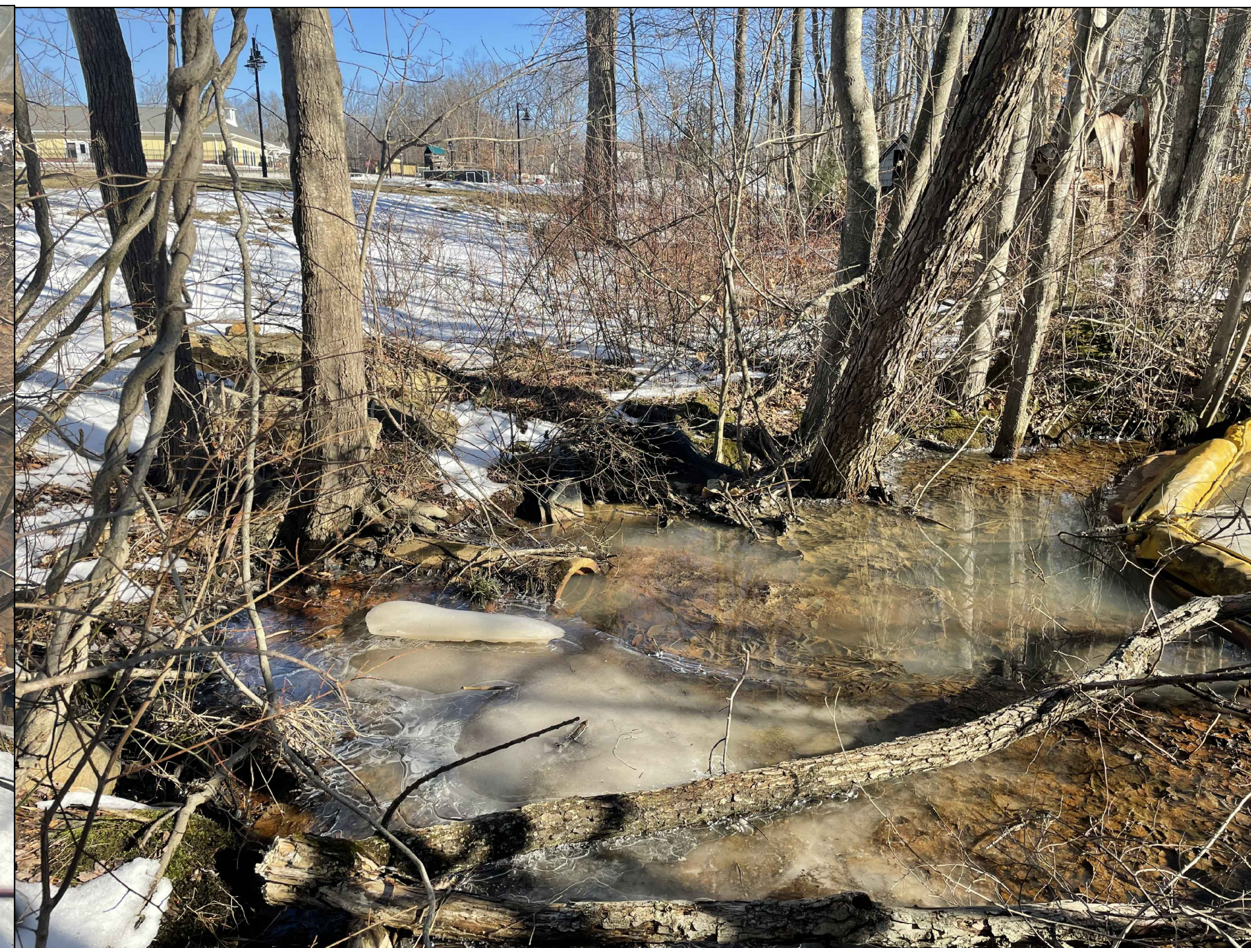
POND AND OUTLET PIPE #1
