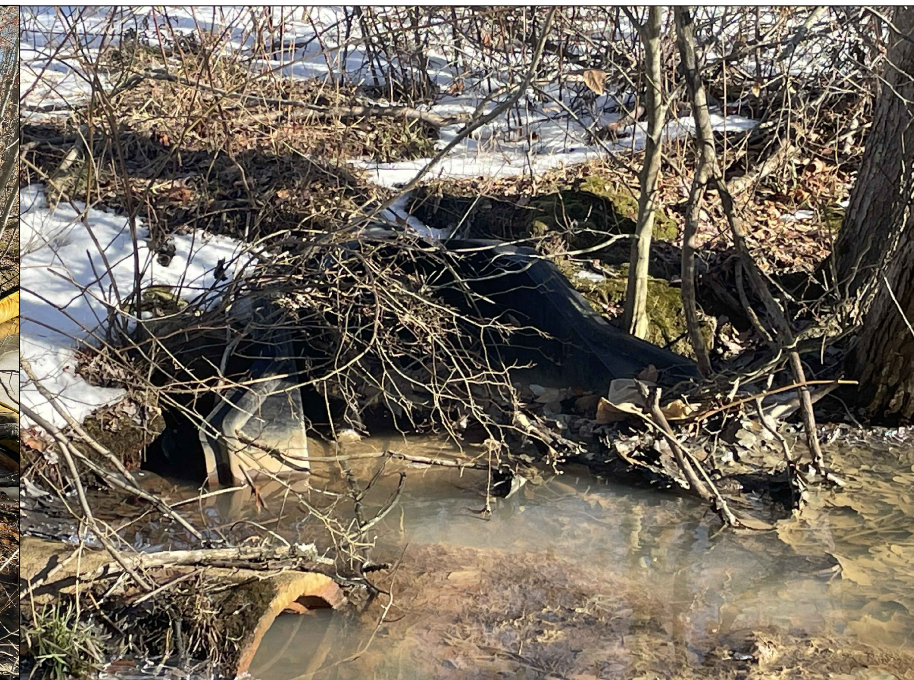
POND AND OUTLET PIPE #2
