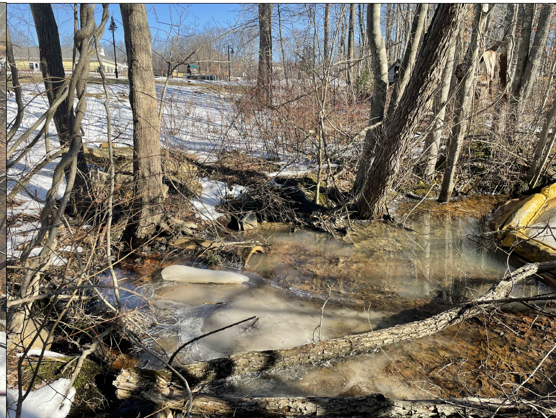
POND AND OUTLET PIPE #1
