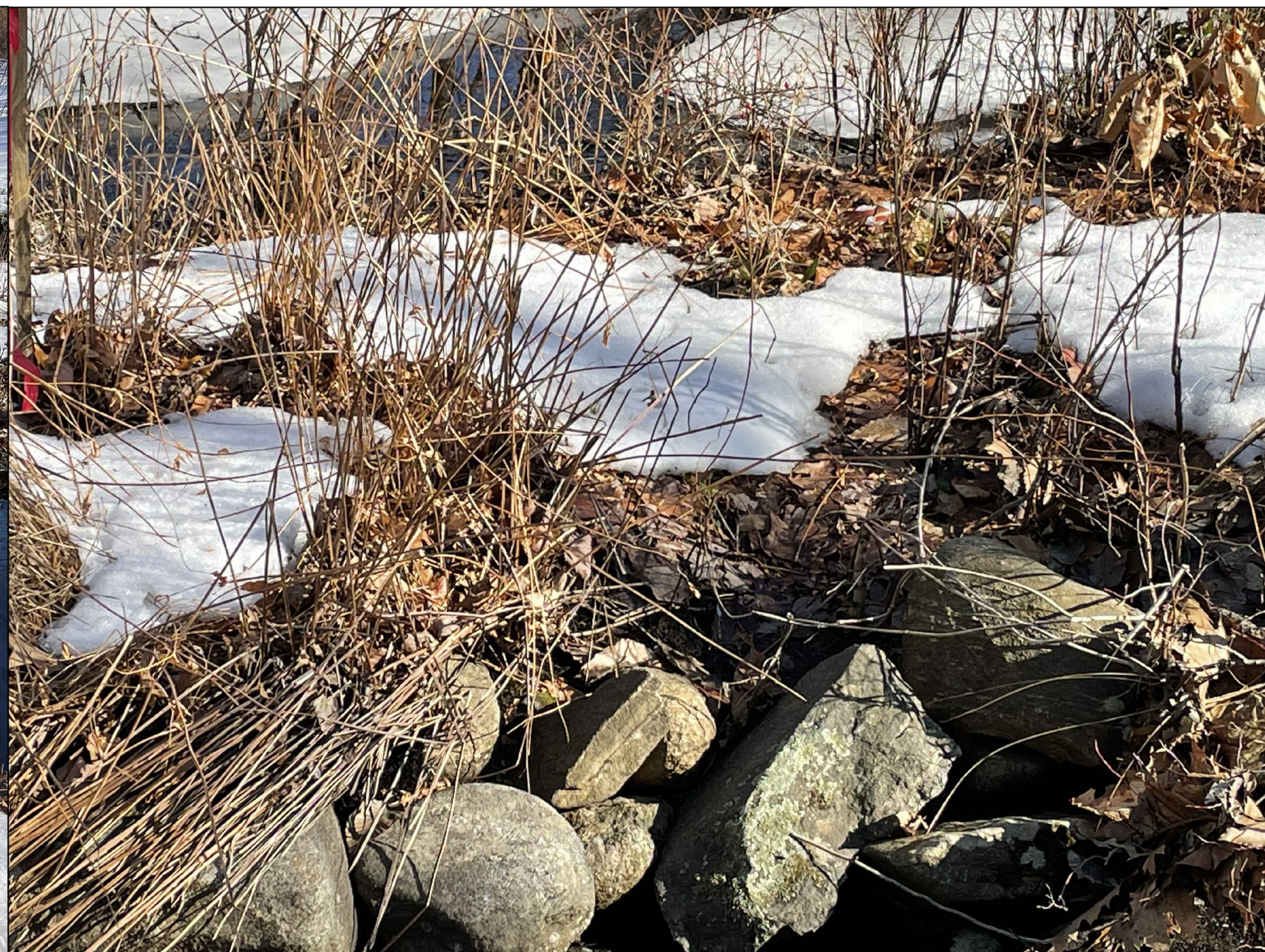
LOCATION WHERE SOIL TO BE REMOVED TO ELEVATION OF TOP OF STONES ON UPHILL SIDE OF SAND BAG BARRIER
