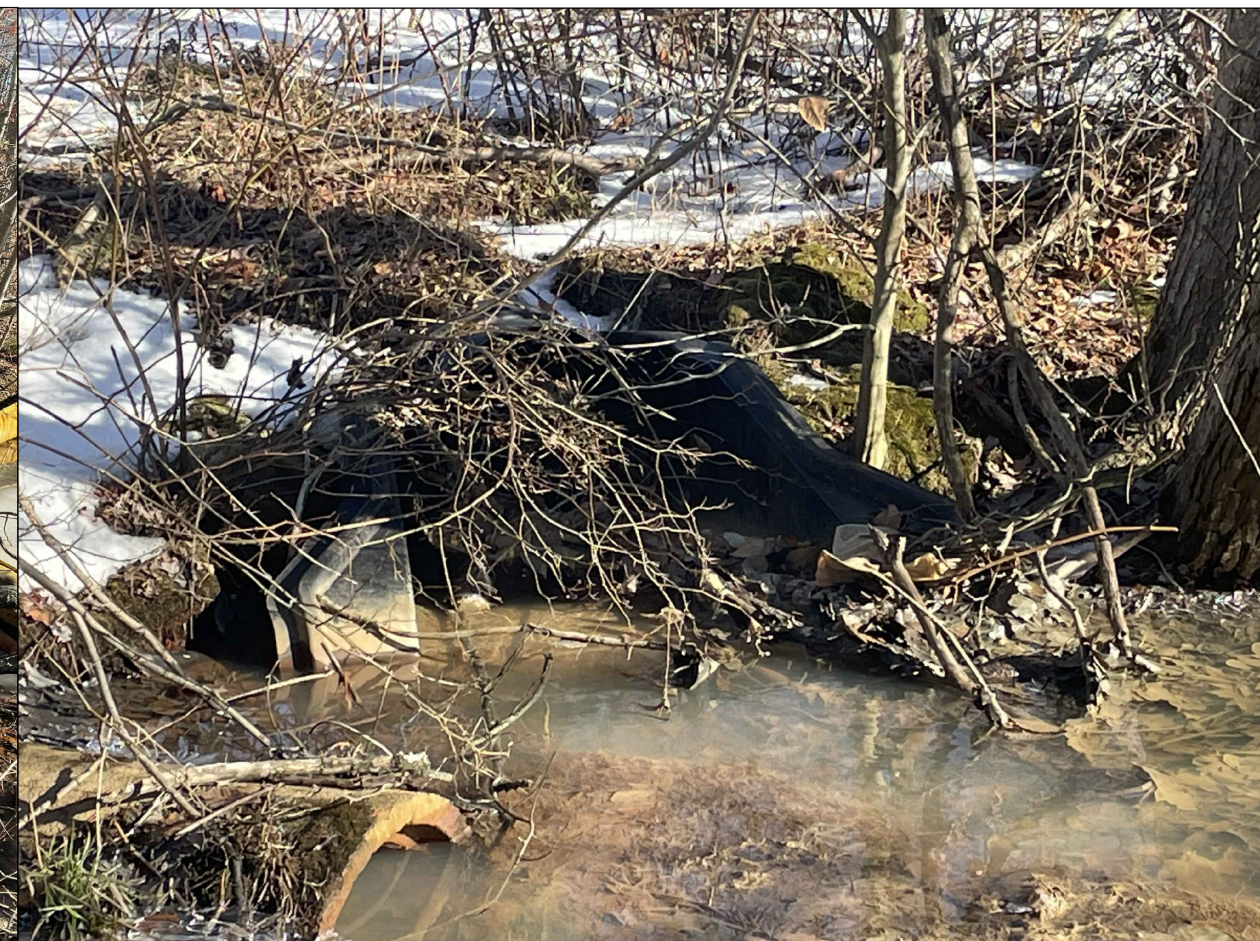
POND AND OUTLET PIPE #2
