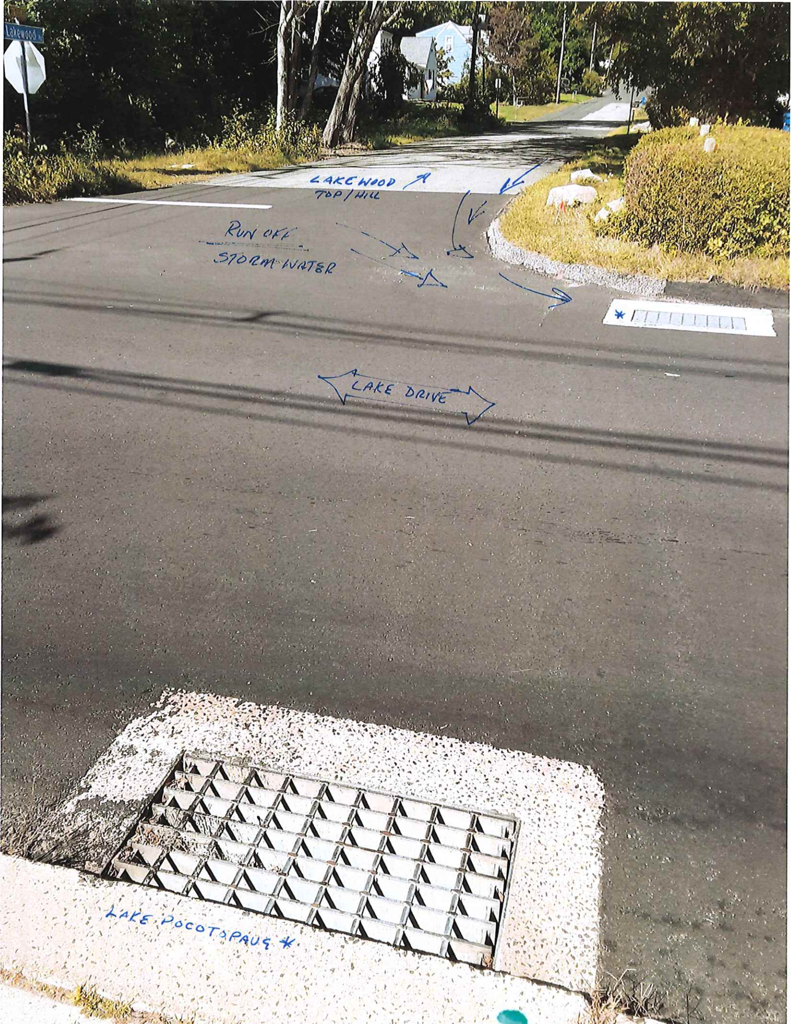
8A ROAD SHOULDER OF LAKE DRIVE - STORM DRAINS - FROM LAKEWOOD RUN OFF
