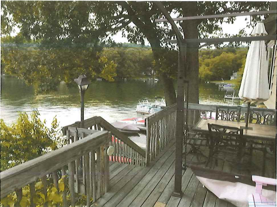
Upper deck midpoint, looking North to upper stair landing 3' x 3'
