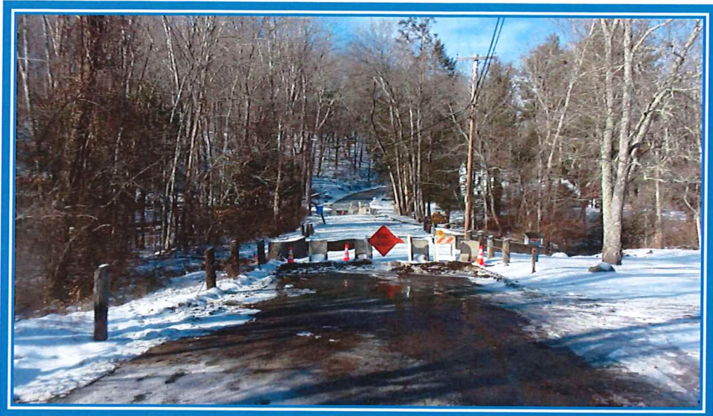
Looking north across Wopowog Road bridge.
