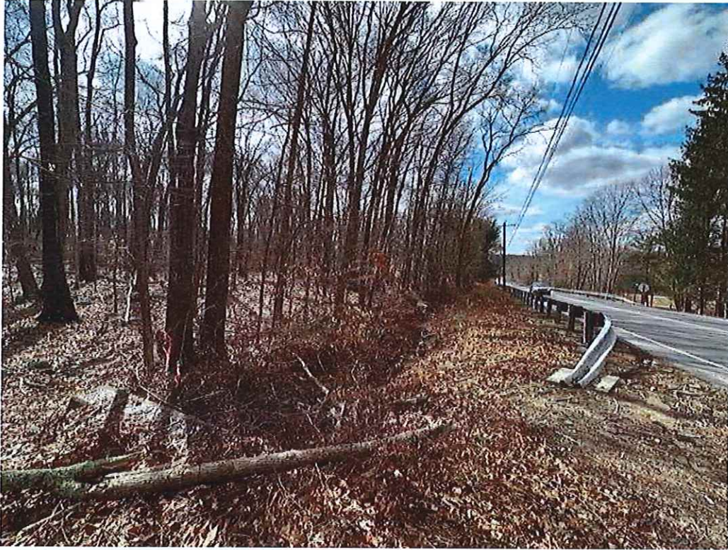
Photo 1: Drainage that runs along the road frontage.
