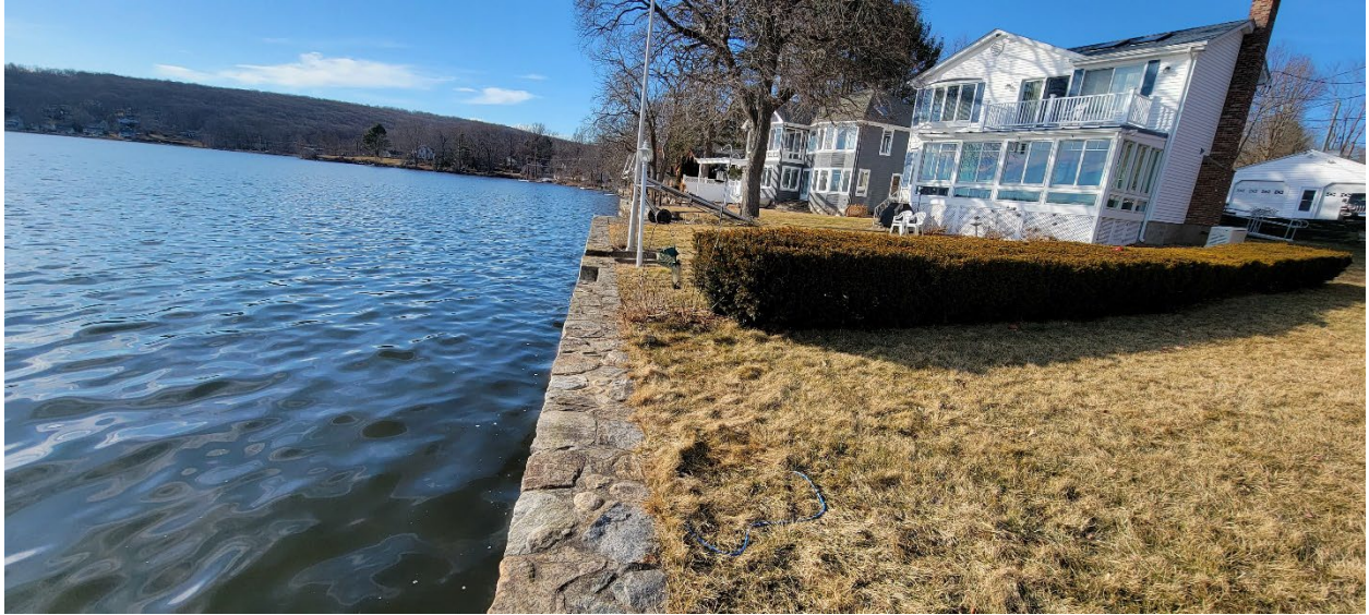
View of Retaining Wall at Shoreline Facing Northwest
