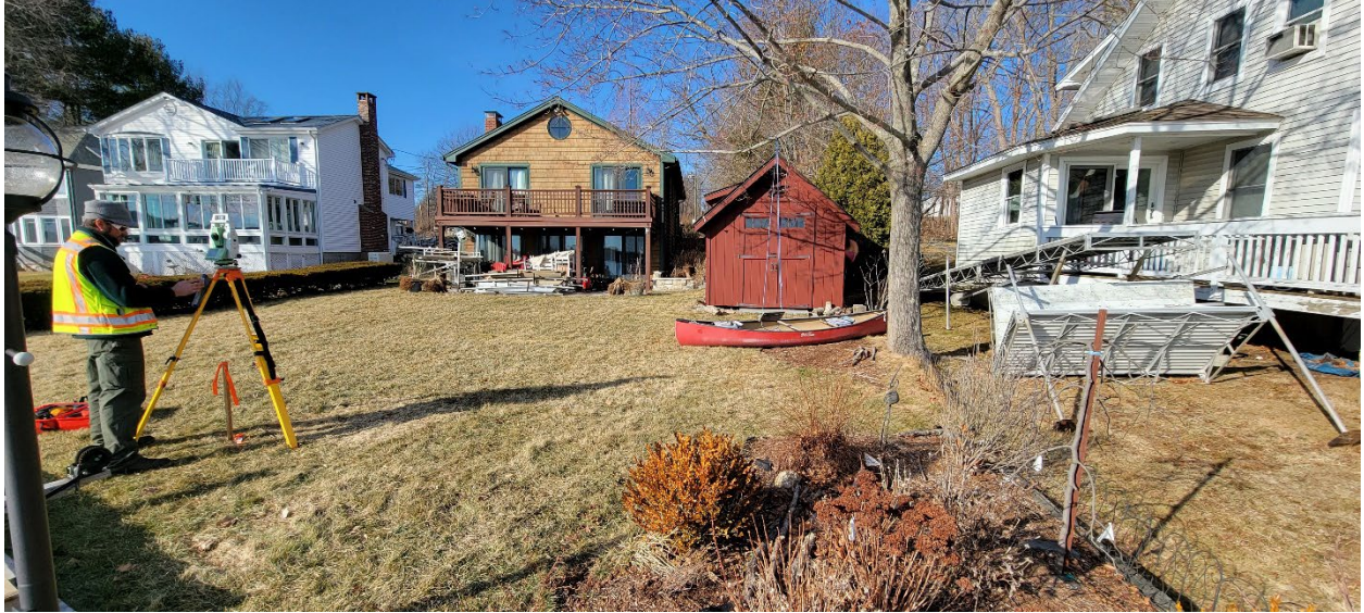
View of Yard Between Existing House and Lake
