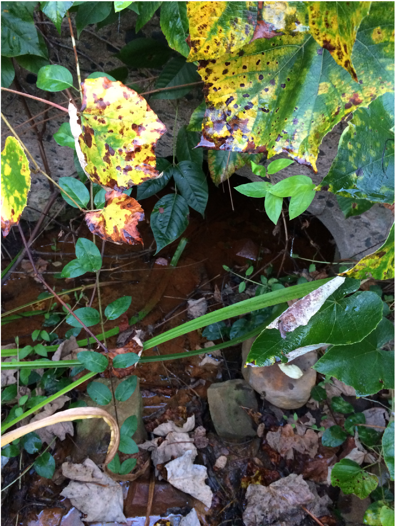
Headwall and 30-inch Culvert Inlet Towards CT Route 66
