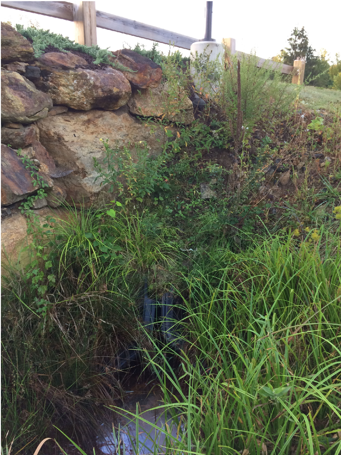
Edgewater Hill Drainage Discharge to Wetlands Adjacent to CT Route 66
