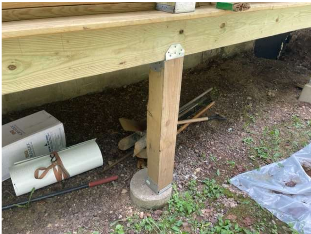
View of column on existing pier.
