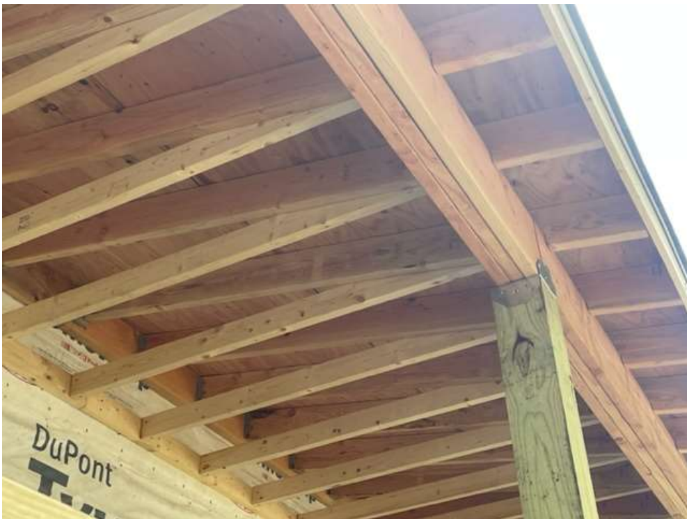
View of roof framing.
