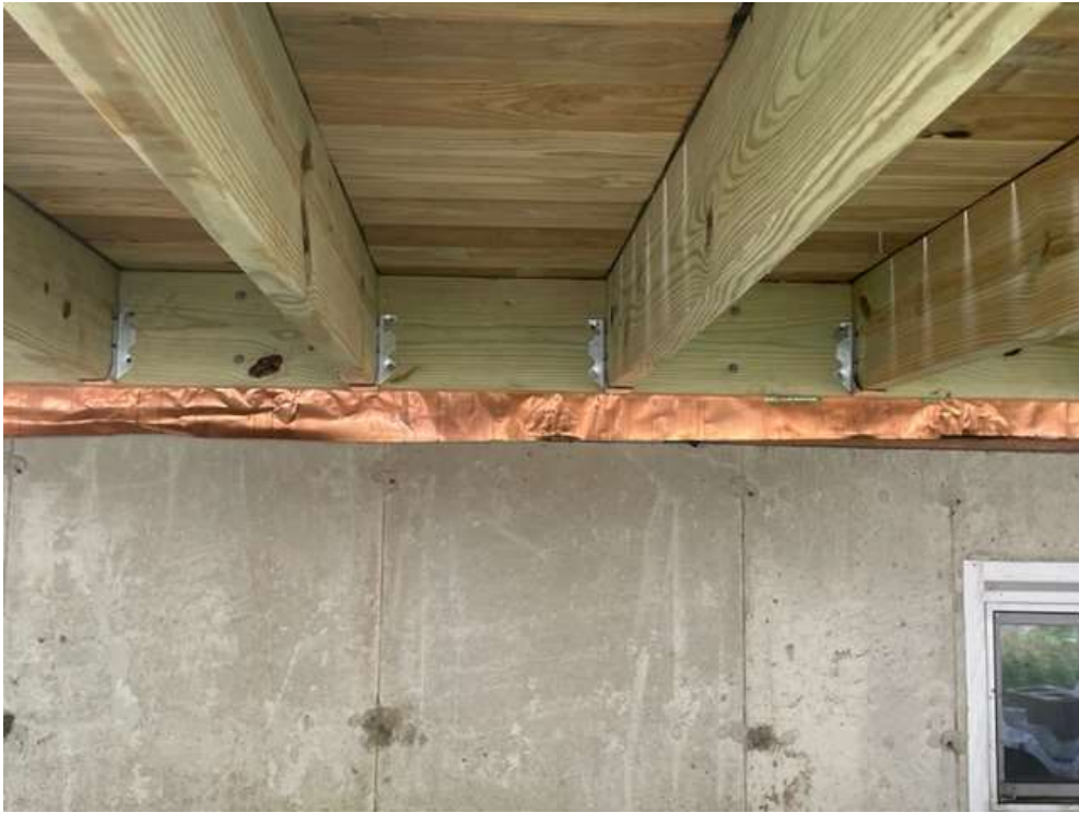
View of ledger with two rows of anchors @ 32".
