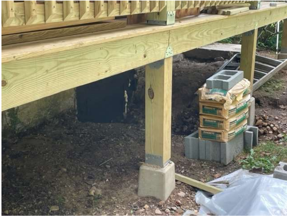
View of columns on precast piers.
