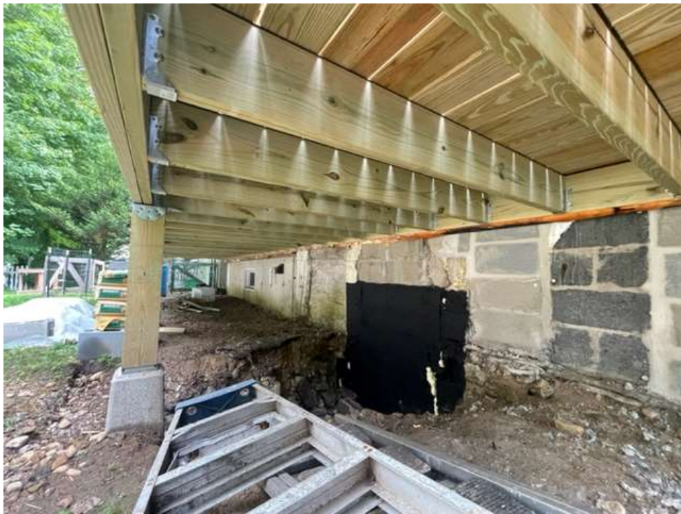
View of floor framing.
