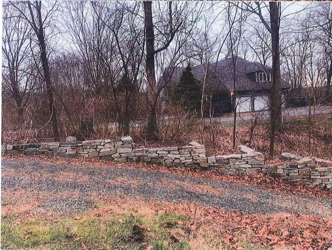
Wall adjacent Kelly Property along the path
