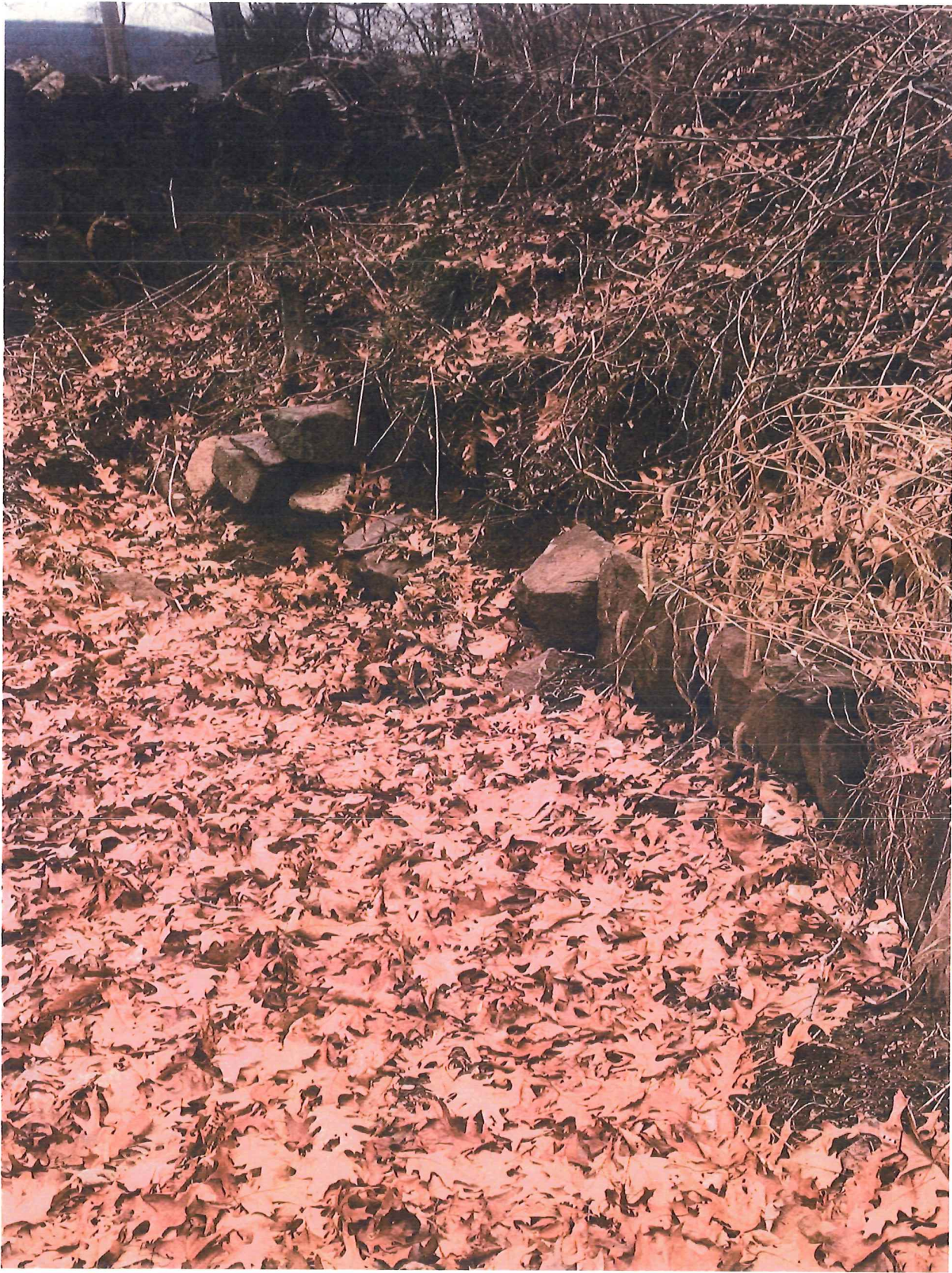
Ice House foundation
