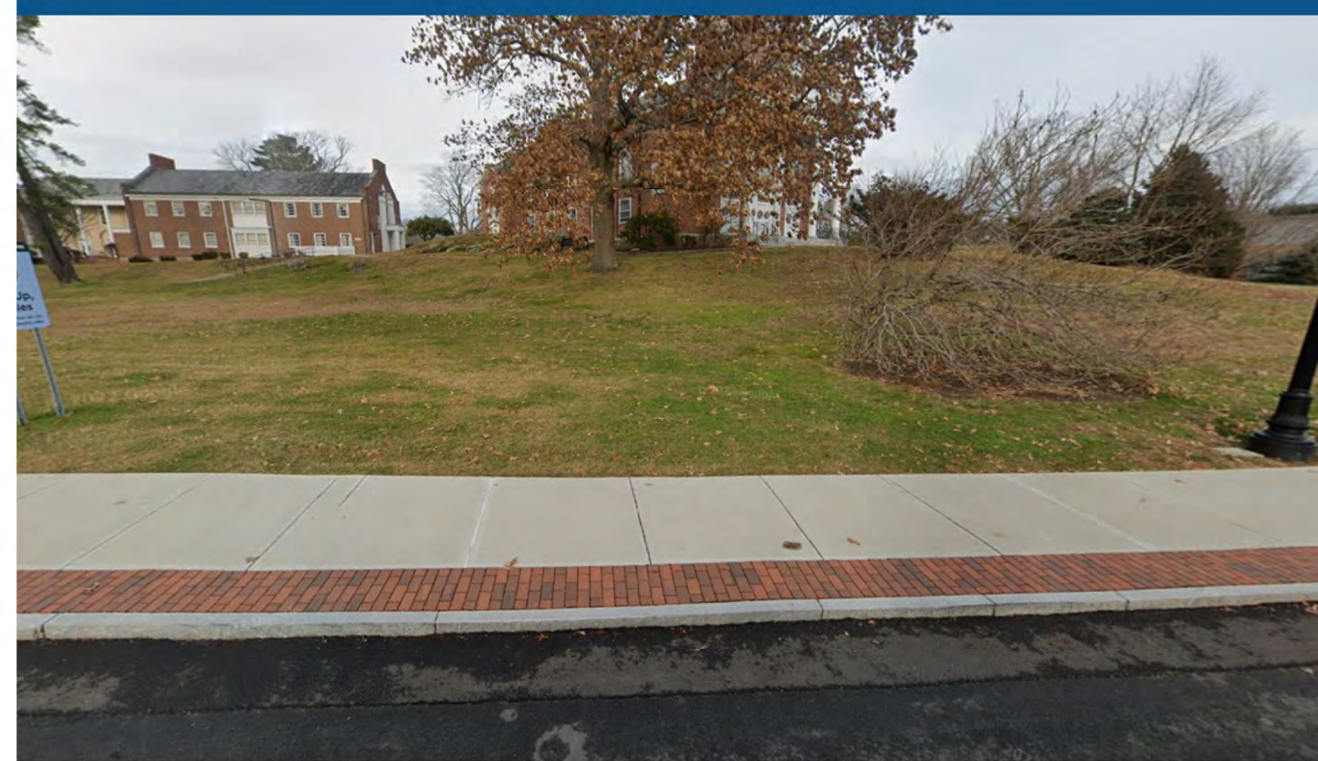
7 BRICK AMENITY STRIP TO BE PLACED BETWEEN CURB AND SIDEWALK (UConn CAMPUS N. EAGLEVILLE RD, MANSFIELD, CT)
