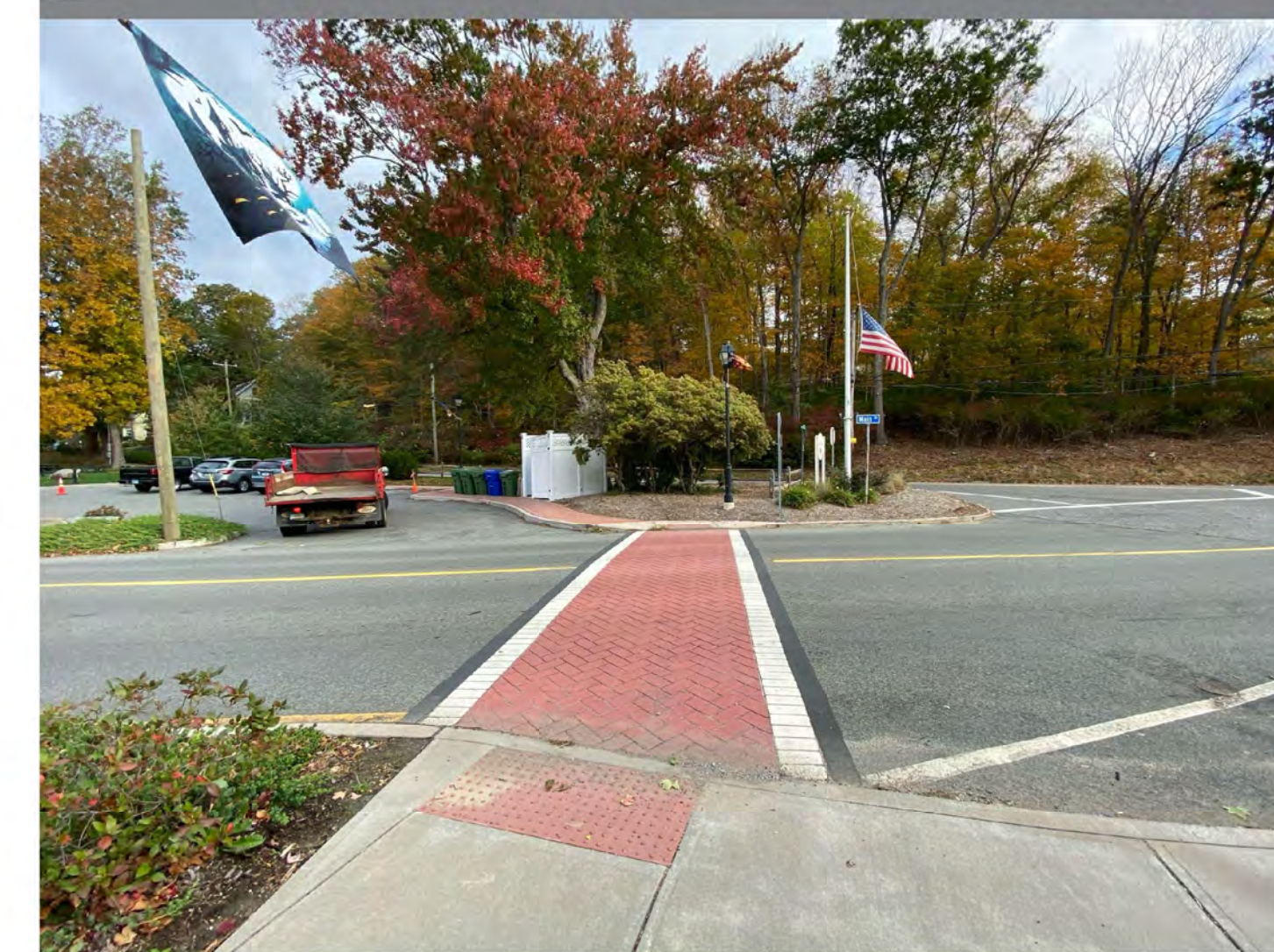
9 THERMOPLASTIC CROSSWALKS (WITH CTDOT COMPLIANT 12" WHITE BANDING) (PHOTO FROM IVORYTON VILLAGE, ESSEX, CT)
