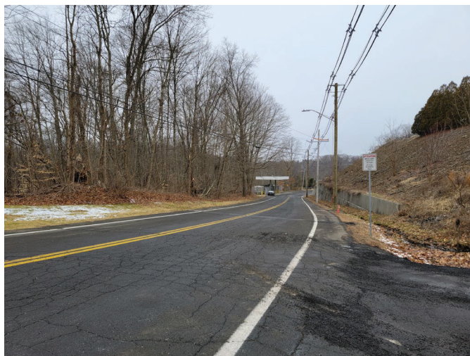
Photo 13 – Proposed Intermediate Pressure Zone Booster Pumping Station Site
