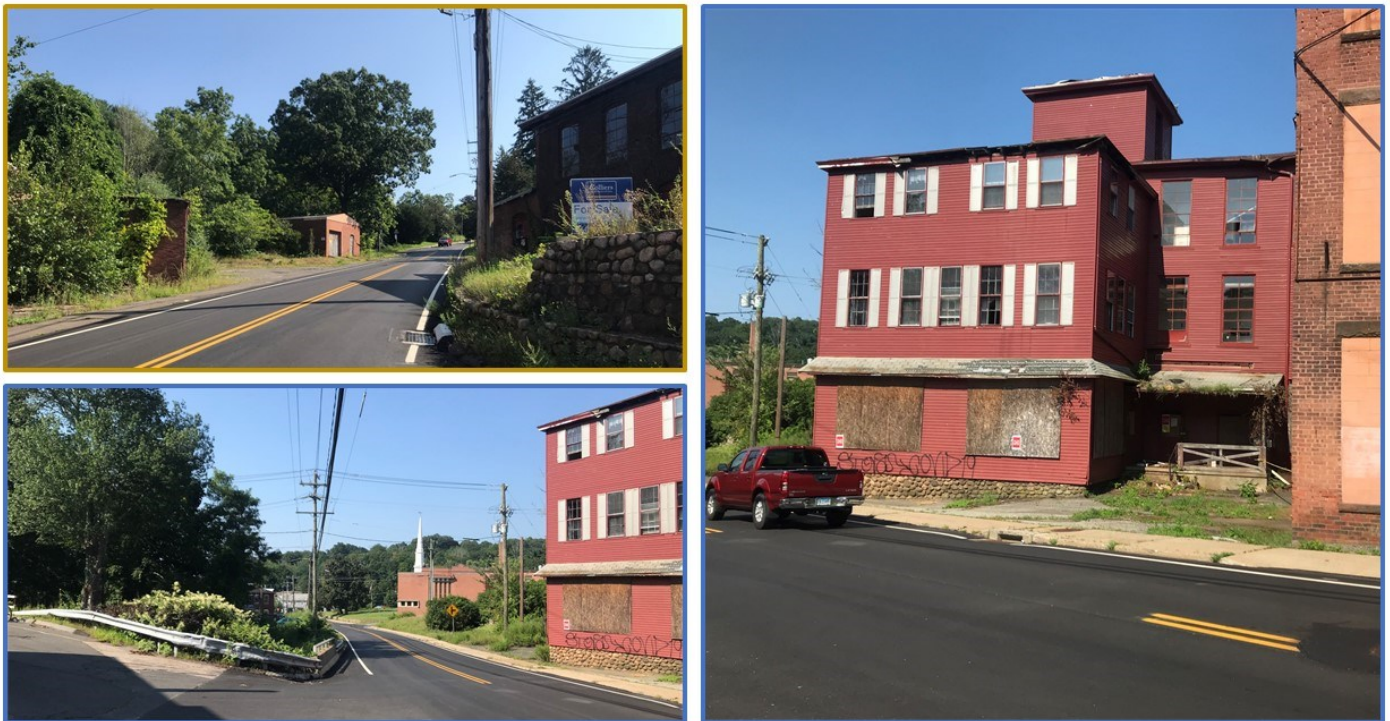
Figure 10: Gateways to the Village Center
