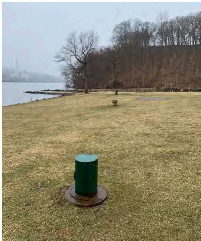
Photo 2: Cobalt Wellfield Existing Conditions
