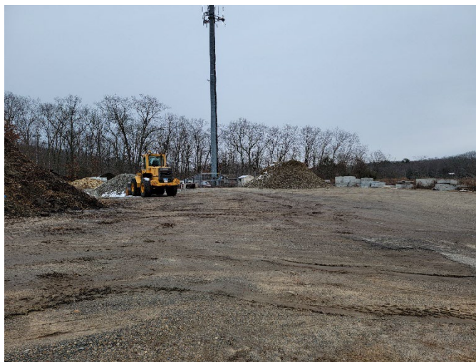
Photo 9 – Proposed Low Pressure Zone Tank Site (Alternative #1, 1 Public Works Drive)
