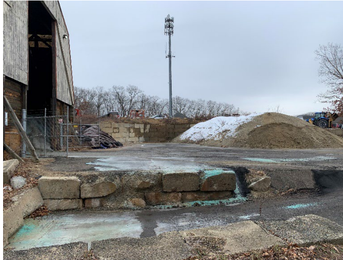
Photo 8 – Proposed Low Pressure Zone Tank Site Existing Conditions (Alternative #1, 1 Public Works Drive)
