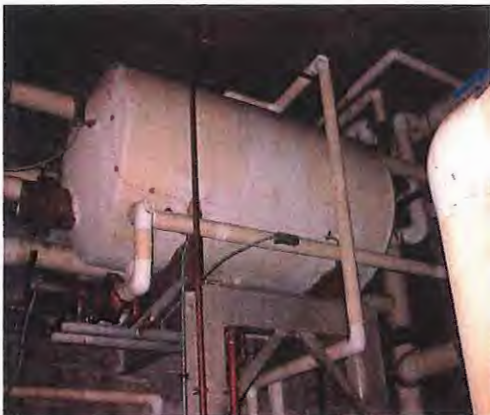
Domestic hot water storage tank.
