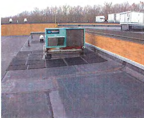
Typical packaged rooftop a/c unit.
