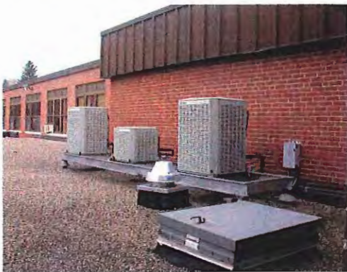
Roof mounted condensing units.
