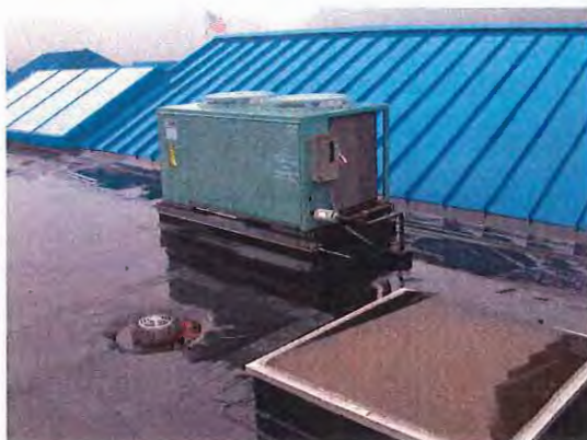
Typical condensing unit.
