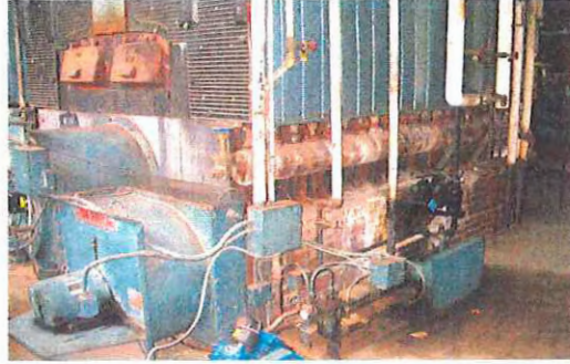
Two Smith section boilers provide heating for the building.
