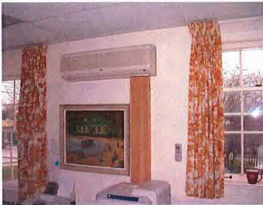
Split DX air conditioner serving the office area.
