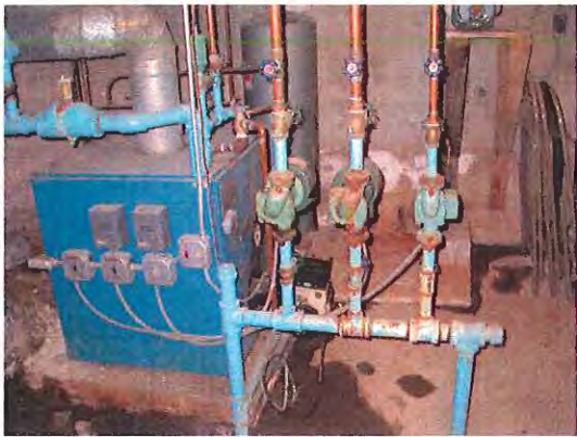
Oil fired boiler located in basement.
