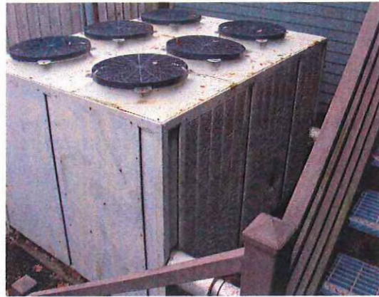
An air cooled chiller is located on the senior graded.
