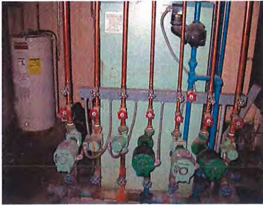
Boiler and in-line hydronic circulators.
