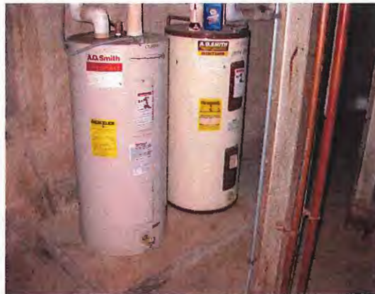
Electric domestic hot water heaters.
