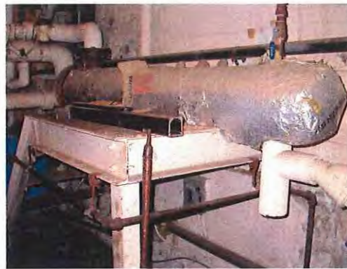
Steam to hot water heat exchanger.
