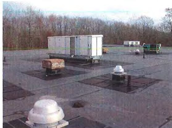
Typical rooftop make-up air handler.
