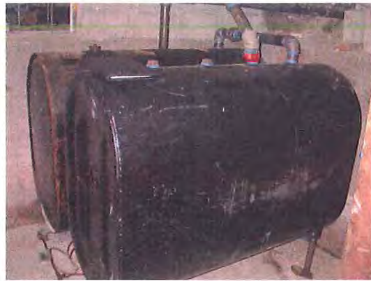
Two 275 gallon fuel oil storage tanks.
