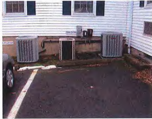
Condensing units serving the air handlers at front of building.
