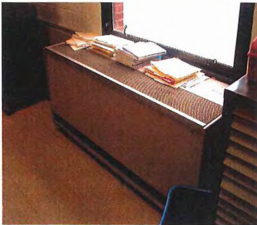
Unit ventilators in newer portion of the school allows outside air into classroom.
