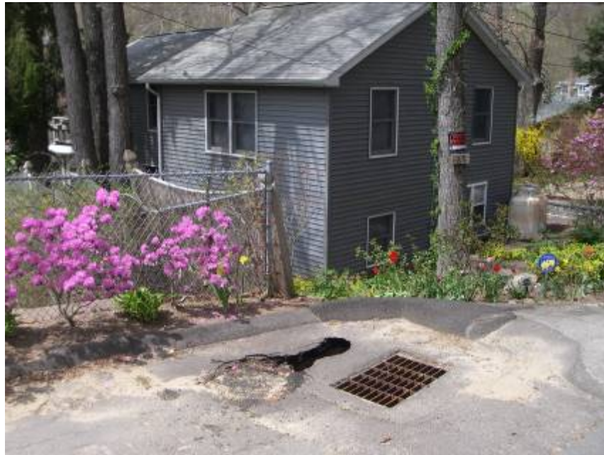
A. Undercut road at Wangonk and Mohigan Trails in subwatershed C
