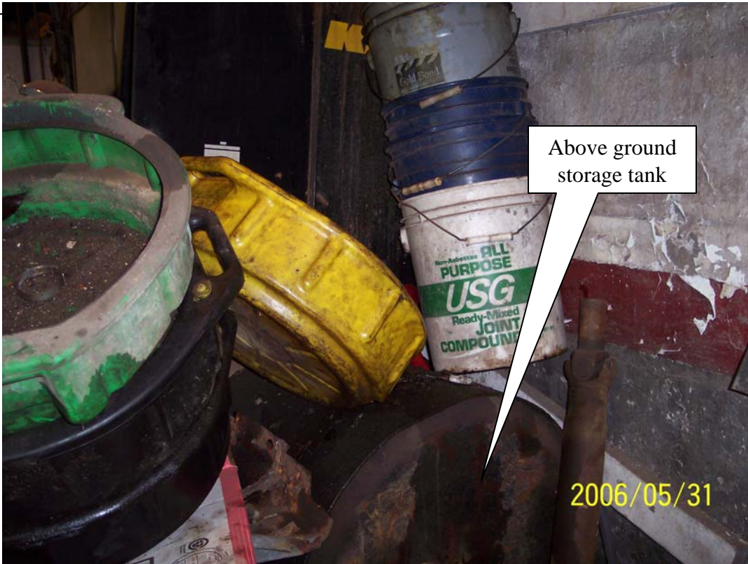
PHOTO: 03 LOCATION: 13 Watrous Street DESCRIPTION: Oil pan draining into above ground storage tank
