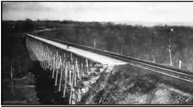
*The Rapallo Viaduct in East Hampton spans Flat Brook on the Airline Railroad. Named for a director of the railroad, it is 1,380 feet long and 60 feet high. It was built out of iron in 1873, and later filled in when trains became heavier.*
