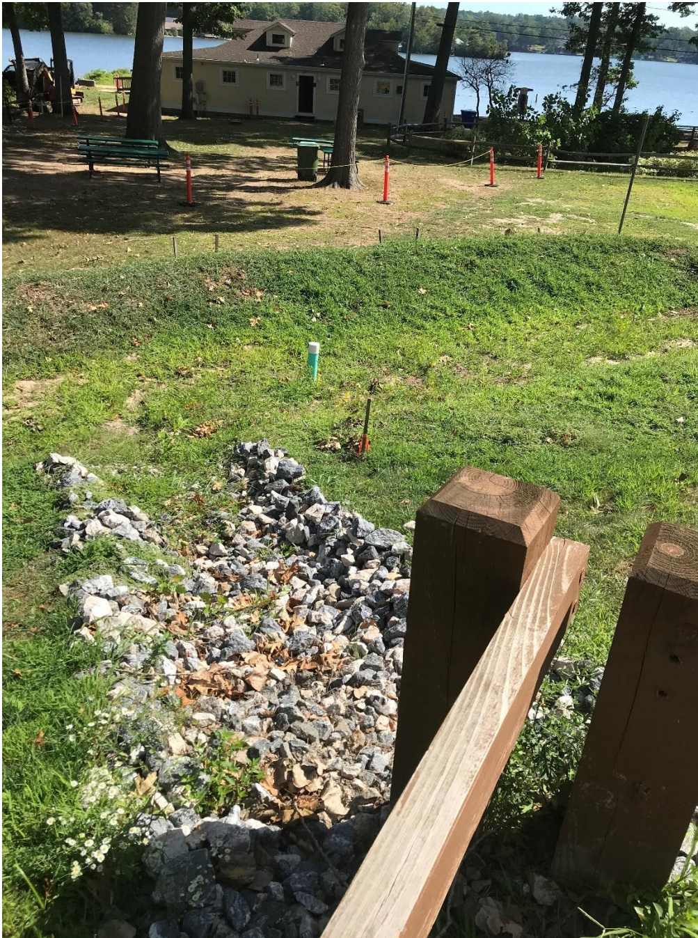
Figure 3 bio retention system #1 Sears Park
