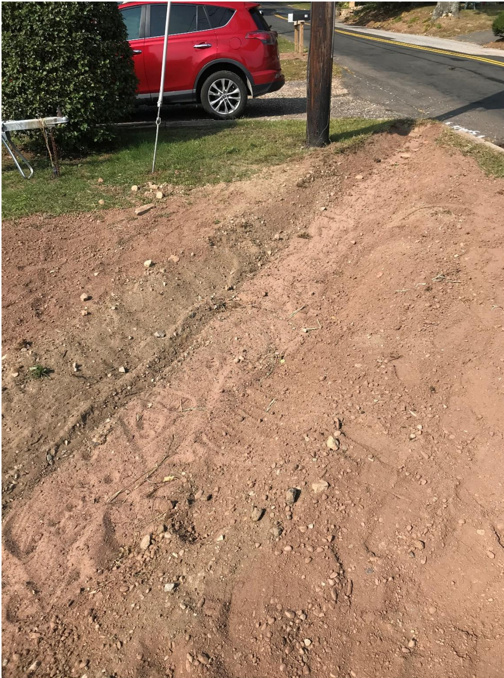
Figure 10 Vegetative swale on Clark hill leading to bioretention system
