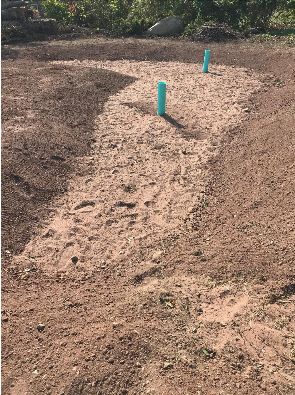
Figure 11 Bioretention system on Clark Hill (pre seed)
