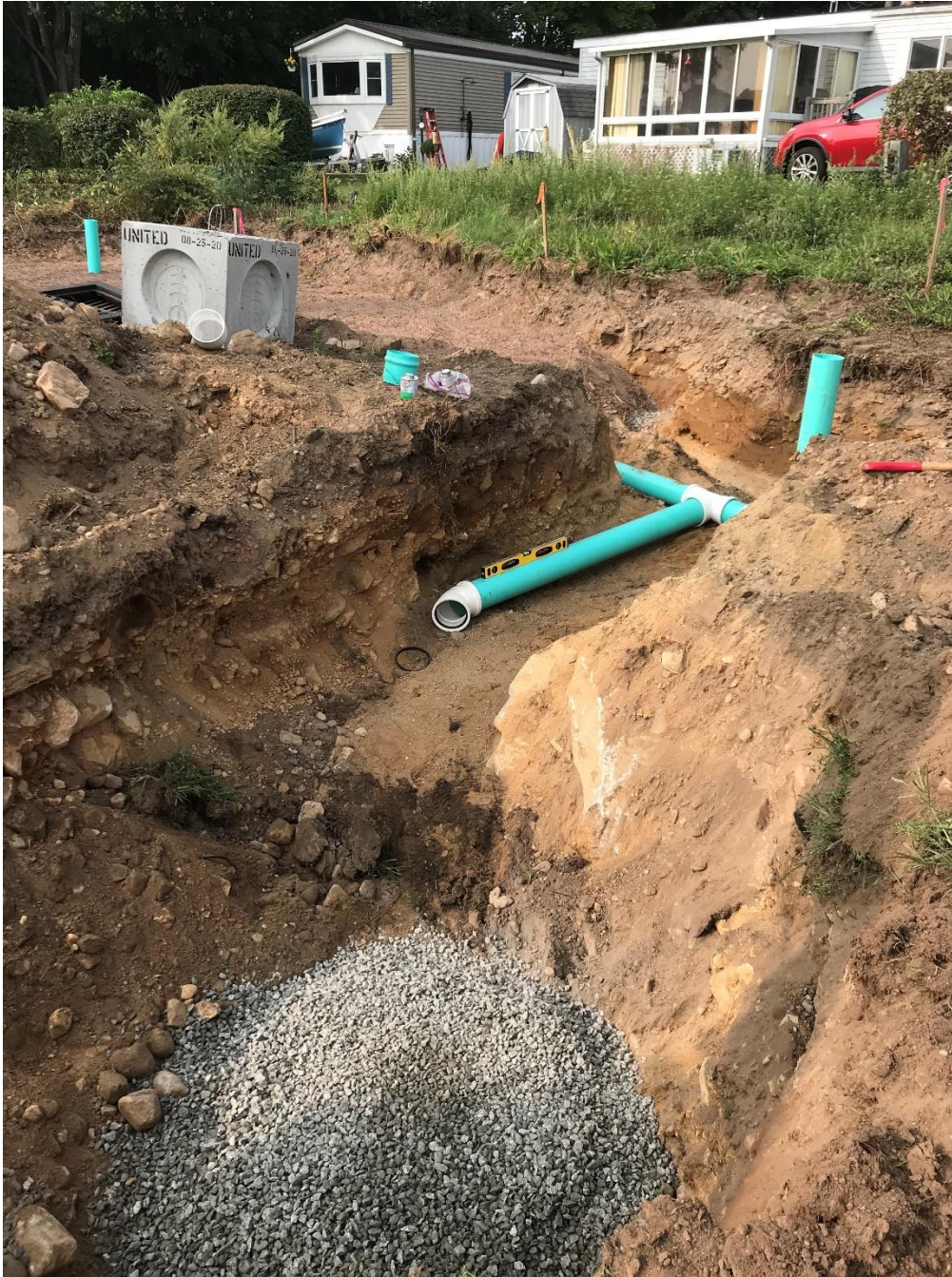
Figure 13 Underground discharge pipes on Clark Hill
